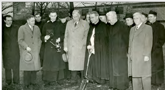
President John J. Long, S.J. (holding shovel), breaks ground for the Fieldhouse on December 8, 1947. Alumni Memorial Fieldhouse would go on to provide 59 years of memories for Saint Joseph's basketball.
